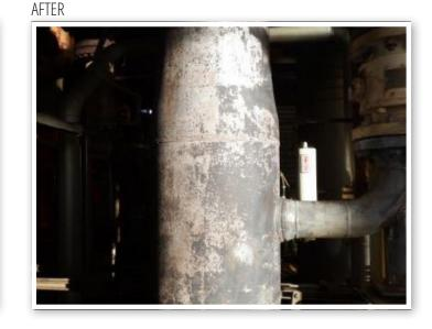
DRY ICE CLEANING REMOVES HEAVY CORROSION AND DEFECTIVE COATINGS FROM PIPEWORK AND ALLOWS FOR MINIMAL DISASSEMBLY, NO DRYING TIME, REDUCED ENCAPSULATION AND WASTE DISPOSAL, WHICH OPTIMIZES THE OVERALL PROJECT TIME.
