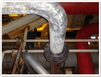
On another similar project, dry ice blasting formed part of a fabric maintenance campaign used by the existing fabric maintenance contractor. This brought nearly 300% gains in productivity and a 65% cost reduction compared with traditional methods.
